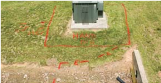
Example of electric transformer, hand dig zone, corridor, lateral
